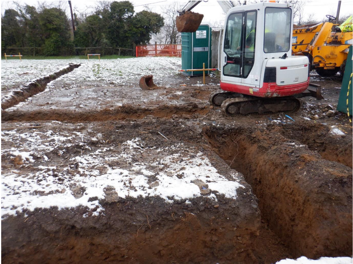
Plate 1. Foundation footings (looking North)
