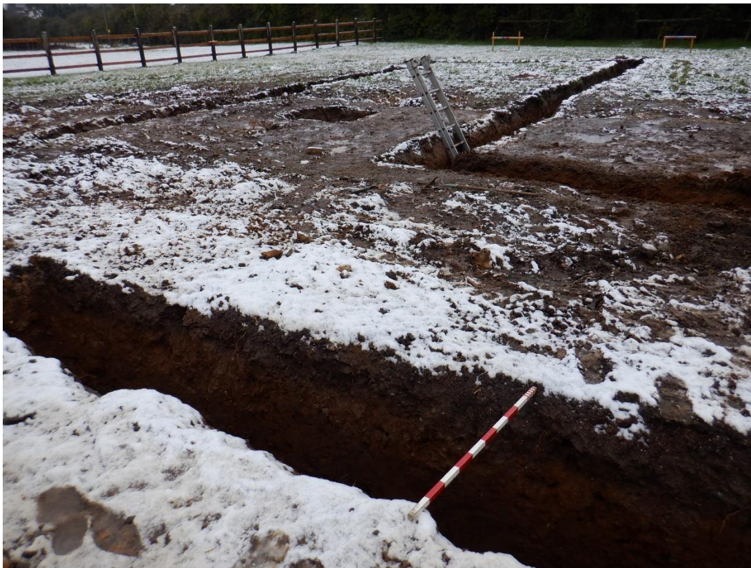
Plate 6. Foundation and drainage trenches (looking NE)
