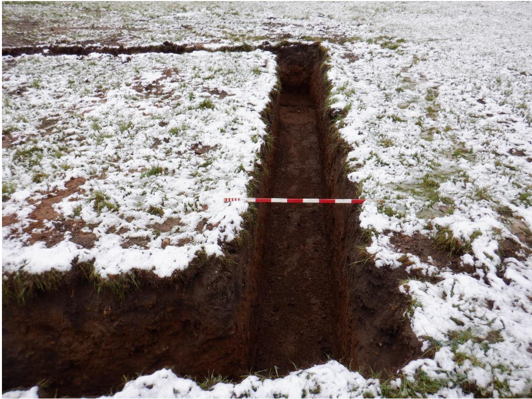
Plate 5. Foundation trenches (looking North)
