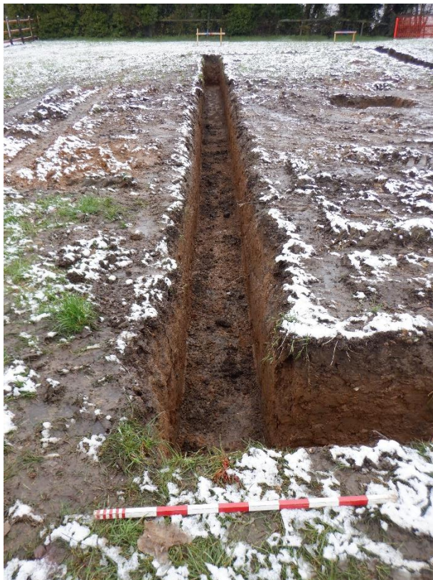
Plate 2. Footings (looking North)
