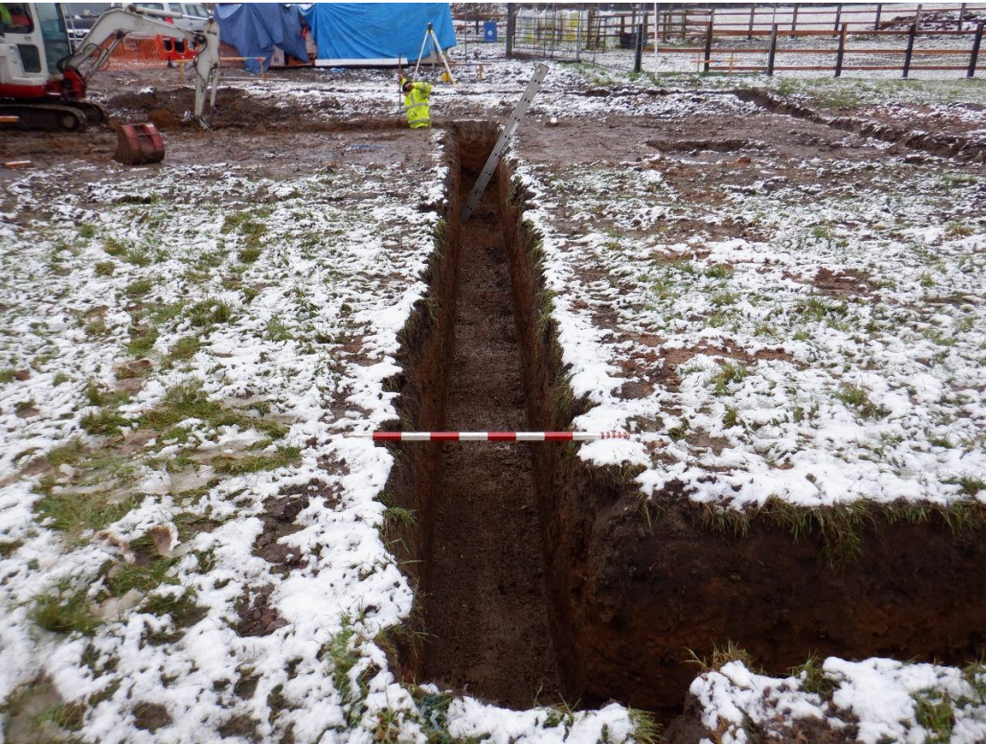
Plate 4. Foundation footing (looking East)
