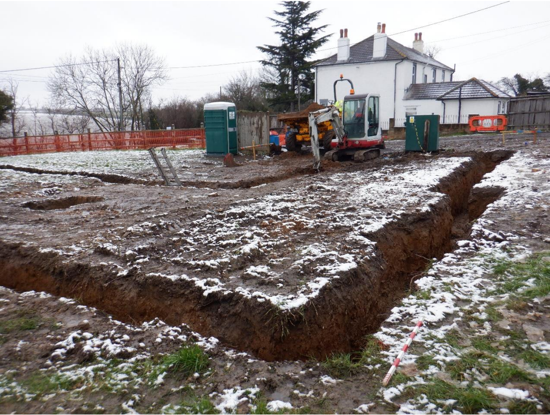
Plate 3. Foundation footing (looking NNE)
